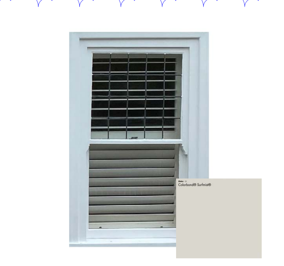
WINDOW FRAMES TO MAGGIE STREET (PAINTED TIMBER, SURFIST)
