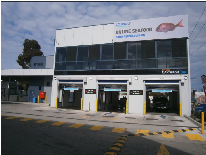
Subject Site from Whitehall Street
