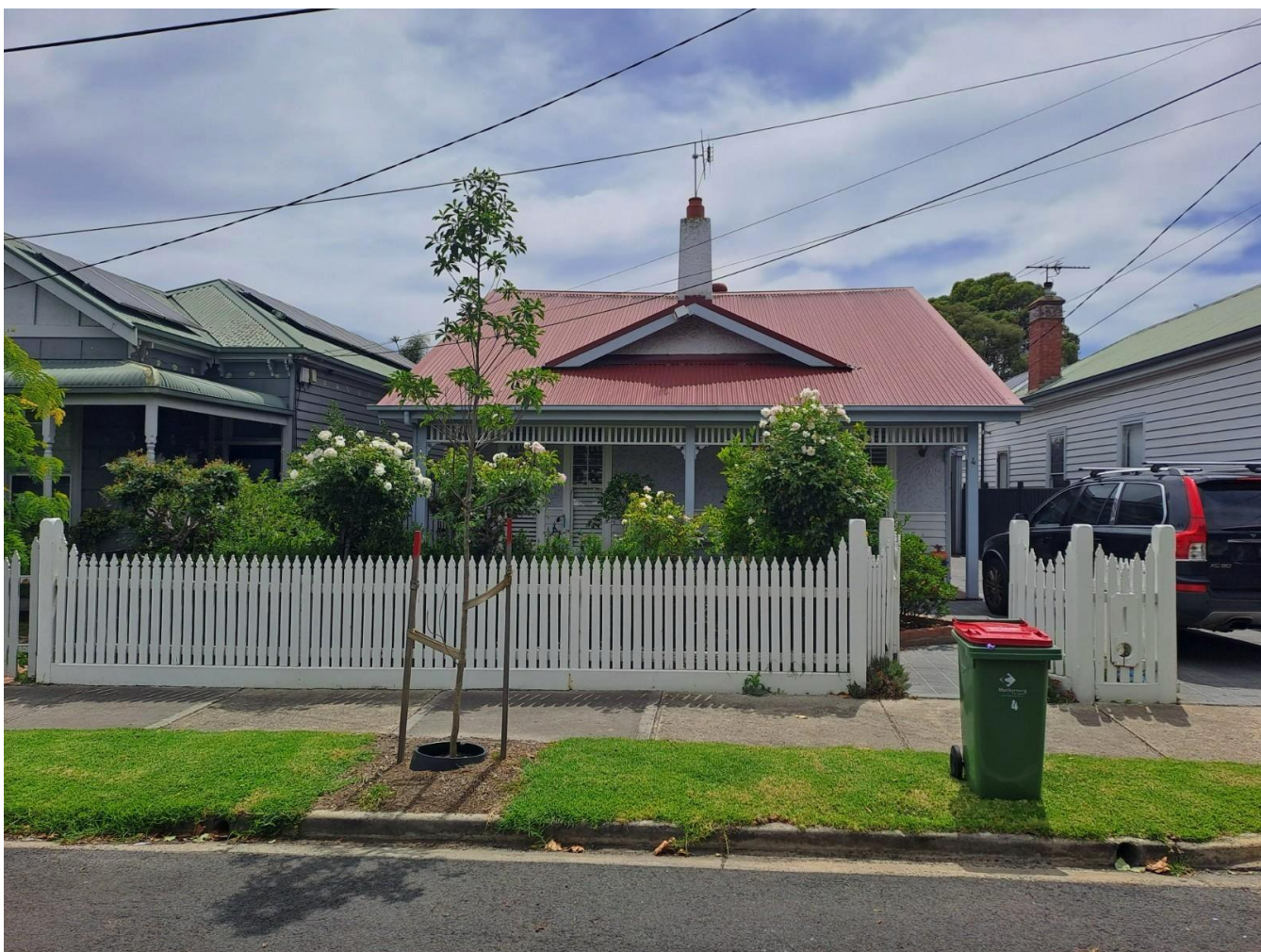
PROJECT SITE 4 WEBSTER STREET
