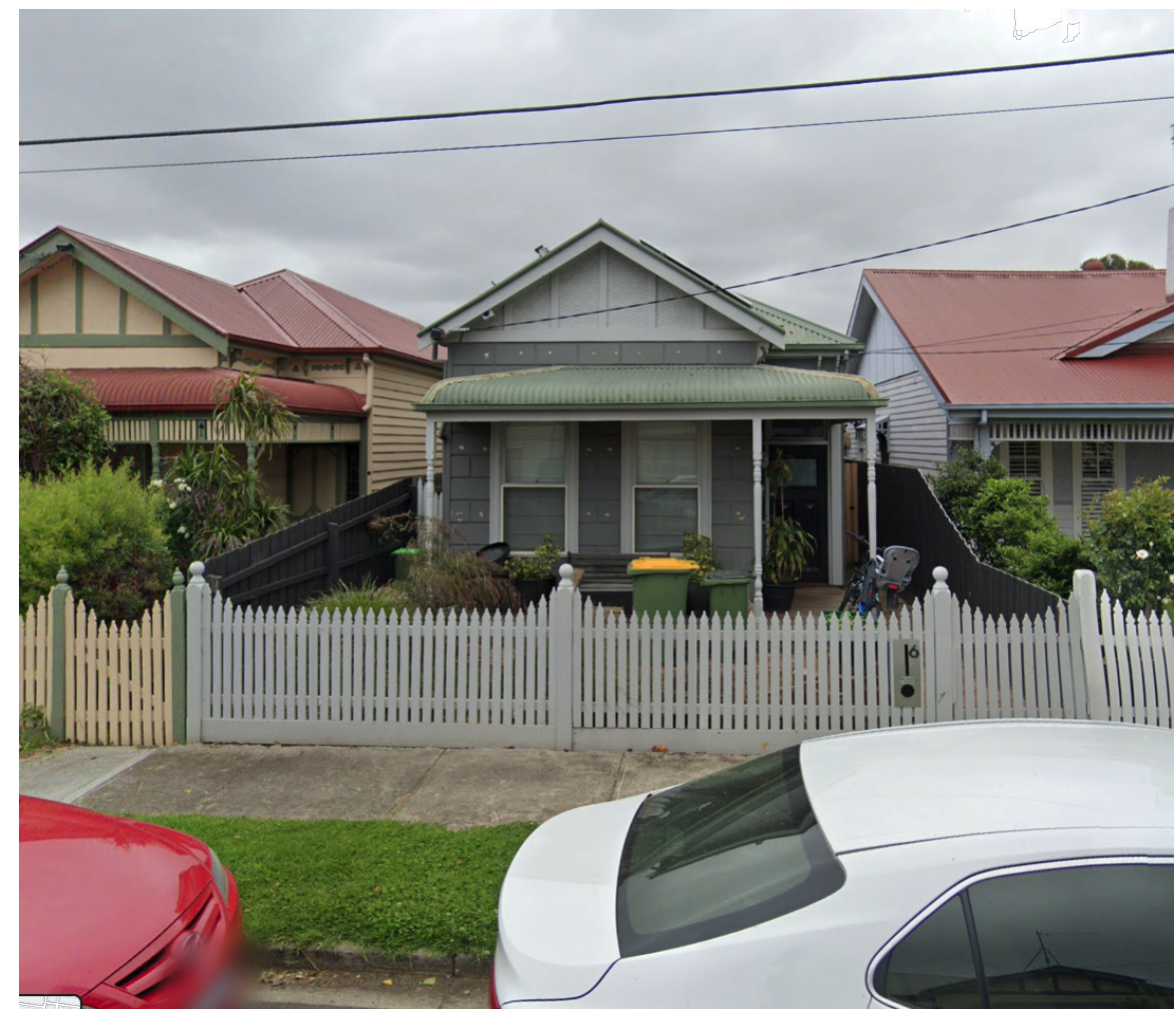
SINGLE STOREY 8 WEBSTER STREET
