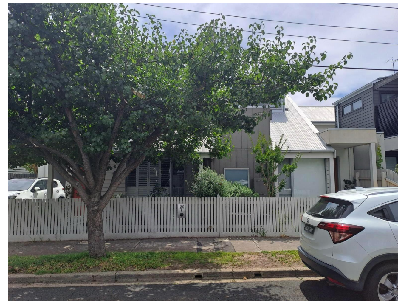
TWO STOREY 2C WEBSTER STREET
