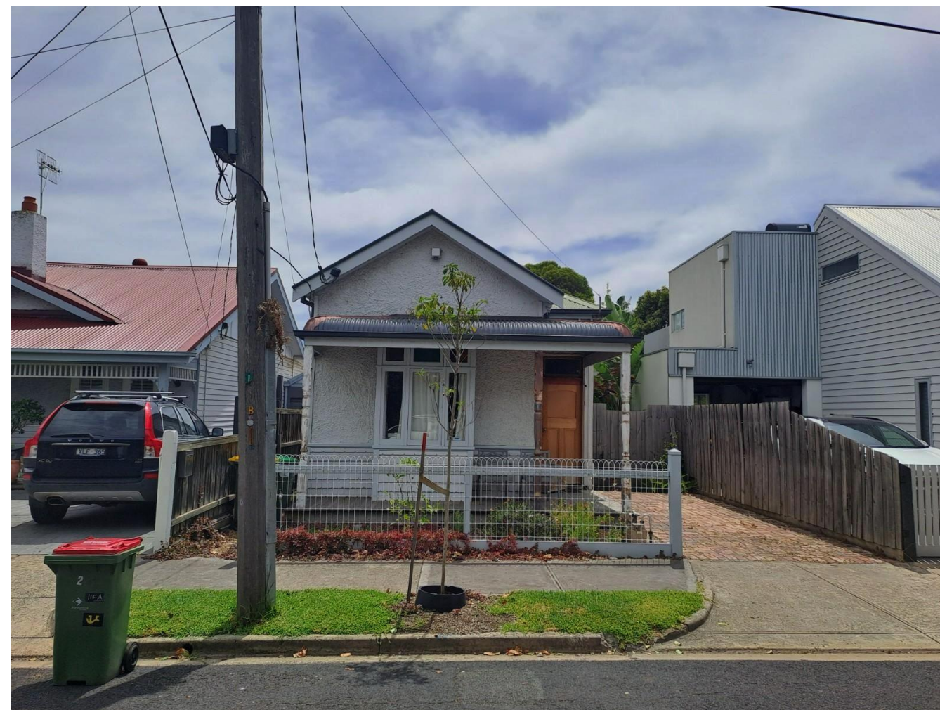
SINGLE STOREY 2 WEBSTER STREET
