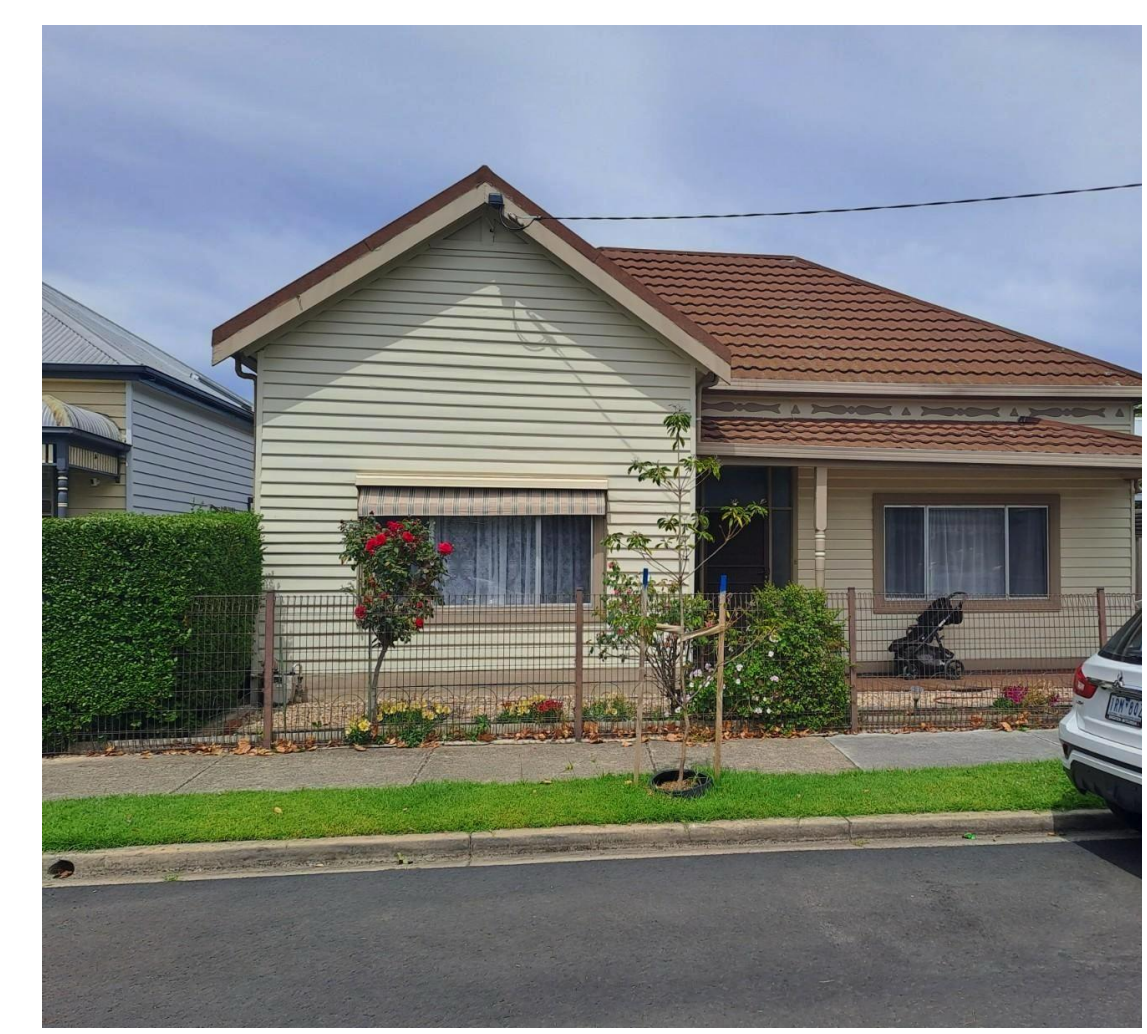
SINGLE STOREY 7 WEBSTER STREET
