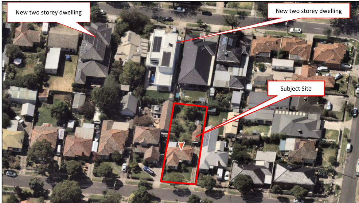
Photograph 1 – Aerial view of site showing the surrounding dwellings
