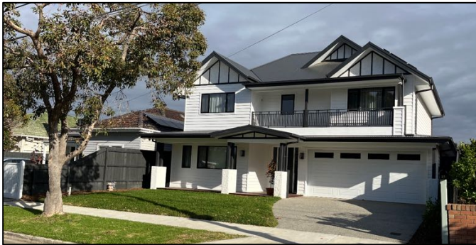
Photographs 9 & 10 – View of the two storey dwellings at 21&22 Rowe Street
