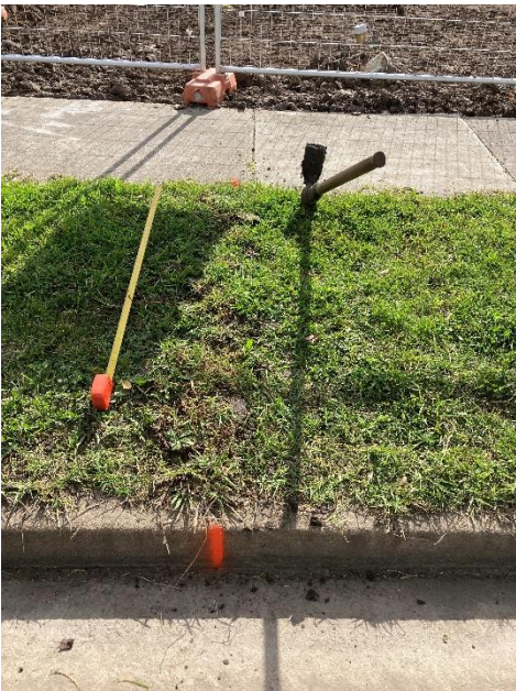
Photo C shows the carefully hand dug root inspection trench, as seen from the south. Illustrating its length and the position of the tape measure in the trench, that was seen in Photo B.
