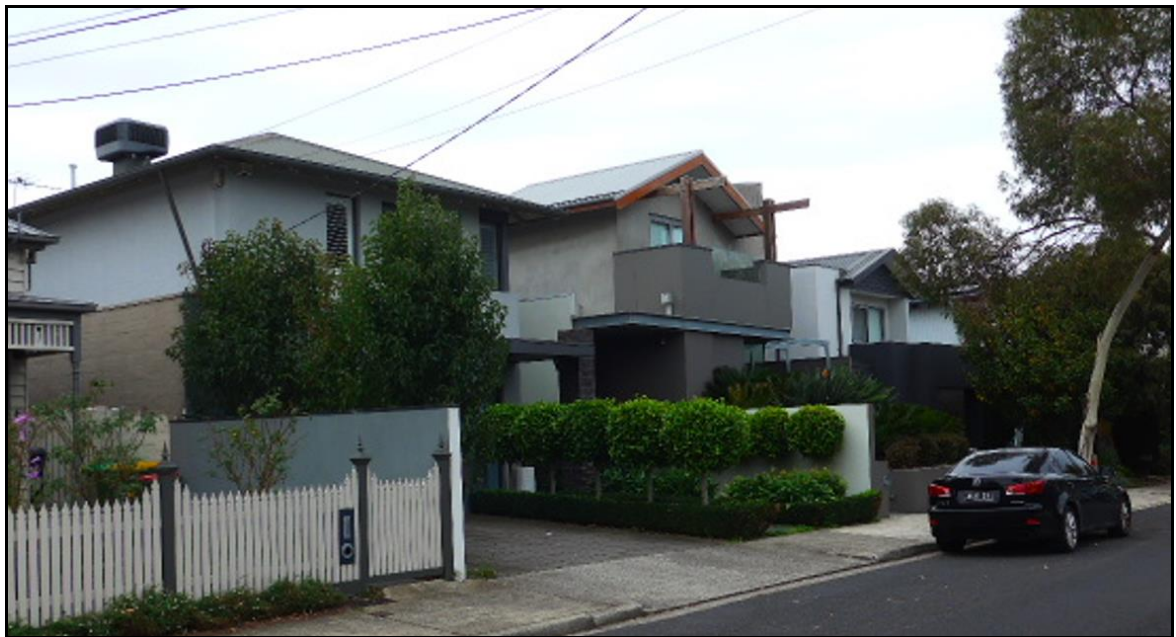
Contemporary style dwellings at eastern end of Castlemaine Street
