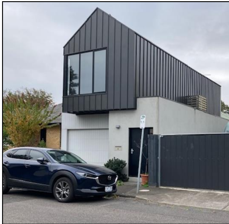
Dwelling at 6 Goulburn Street
