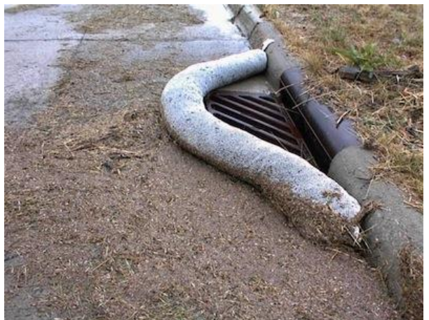
Figure 4 - Sediment Trap
