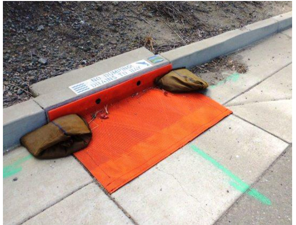
Figure 2 - Sediment Trap
