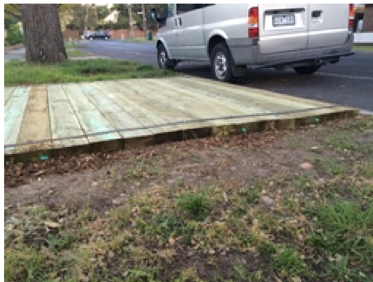
Example of rumble boards used adjacent a street tree.
