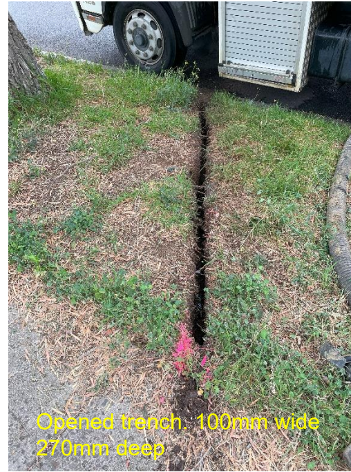
Trench excavated at 2m from trunk centre to middle of splay
