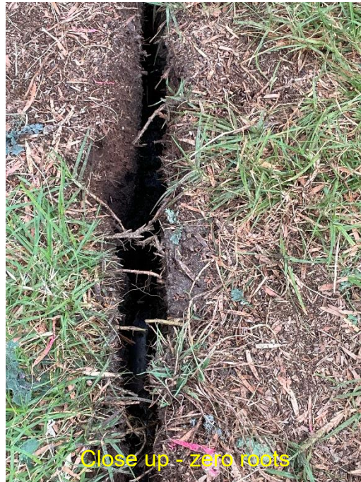
Trench excavated at 2m from trunk centre to middle of splay
