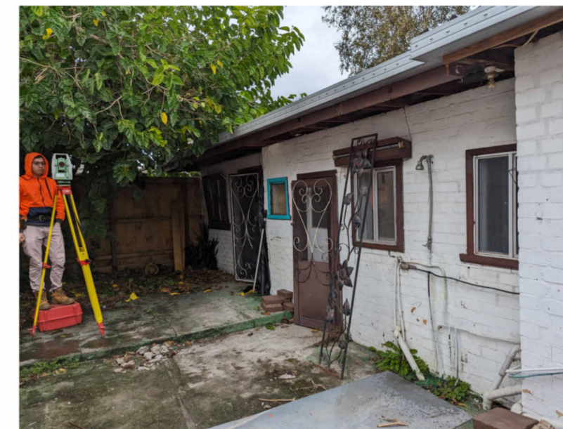
REAR YARD - SHED AND L'DRY / BATH AREA
