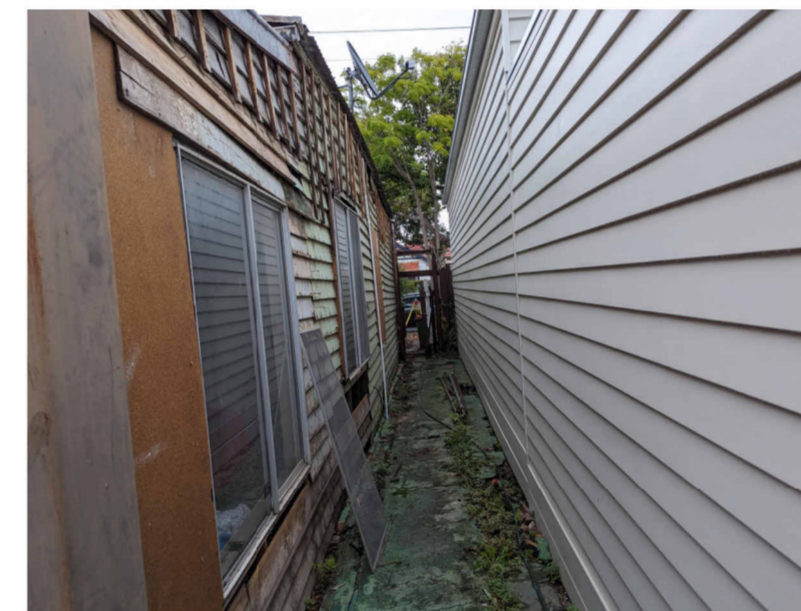
SIDE ACCESS (NORTH OF PROPERTY)
