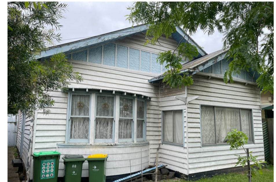
EXISTING FRONT FASCIA/GUTTER ETC. TO BE REPLACED LIKE FOR LIKE DUE TO POOR CONDITIONS EXISTING FRONT NORTH SIDE METAL ROOFING TO BE REPLACED WITH ZINC ROOFING TO MATCH THE EXISTING FRONT SOUTH SIDE ROOFING DUE TO POOR CONDITIONS
