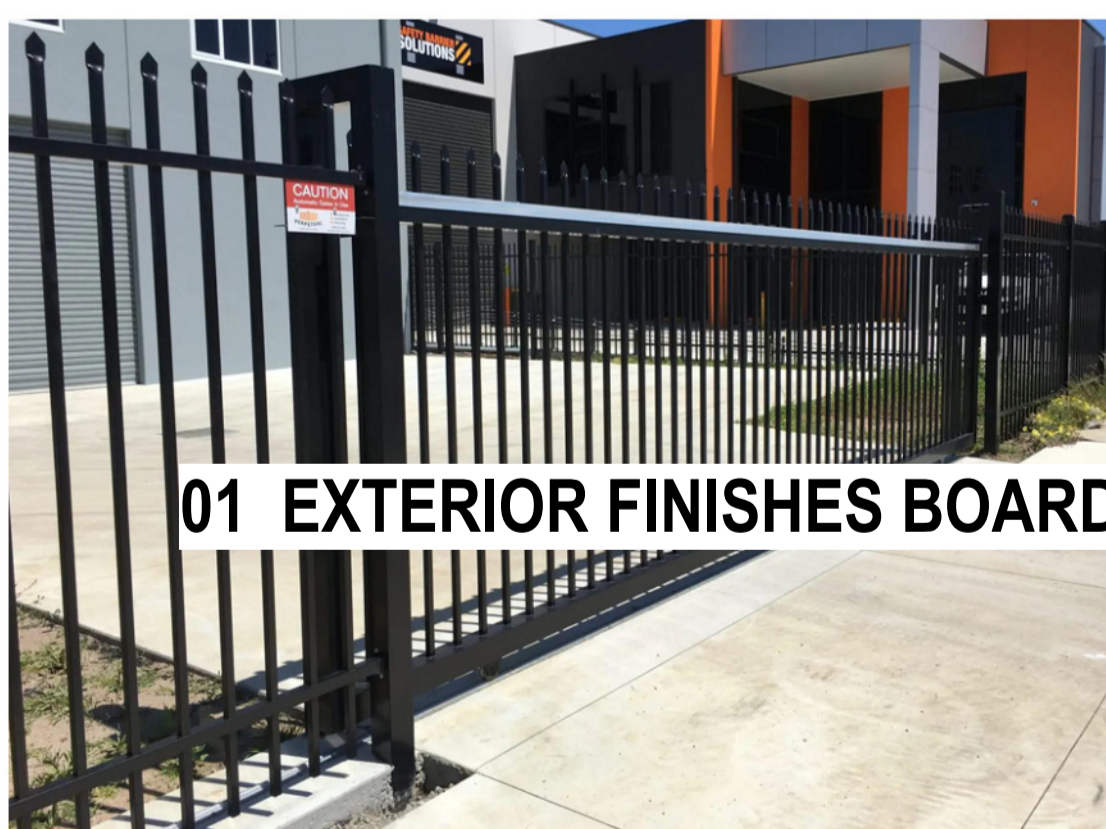
CAR PARK SECURITY FENCE & GATE POWDER COATED METAL PICKETS/FRAME.
