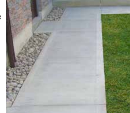
Example of broom-brush concrete by Thundercrete
