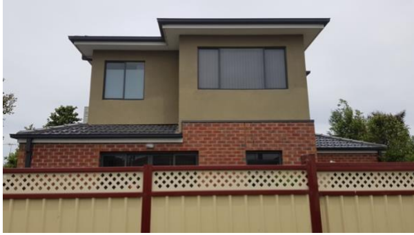
Figure 28 Rear of 12 Gwelo Street
