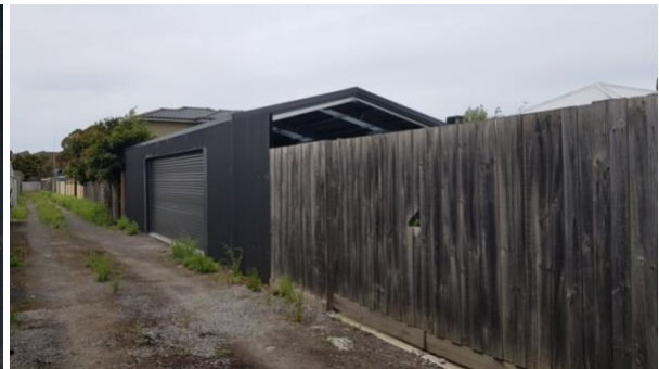
Figure 25 Rear of 16 Gwelo Street (opposite to subject site)
