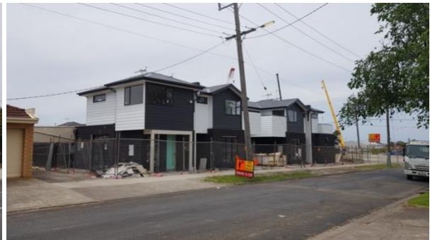
Figure 49 24 Indwe Street (Bizana Street side)
