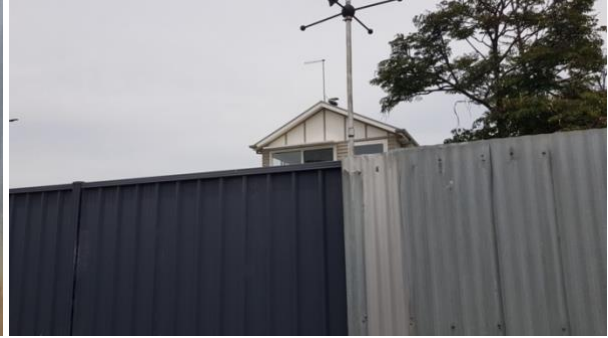
Figure 23 Rear of 20 Gwelo Street
