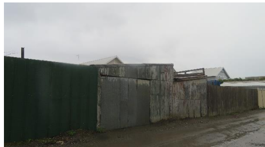
Rear of site (from lane). Note: garage opening in centre
