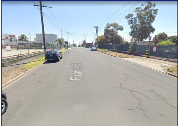
Figure 11: Francis Street, east of Whitehall Street – view west
