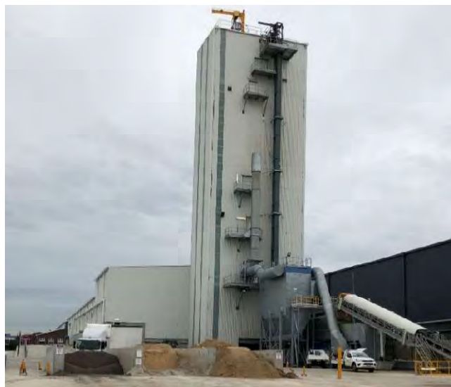
Figure 8: The existing raw material drying, mixing and bagging plant and baghouse stack.
