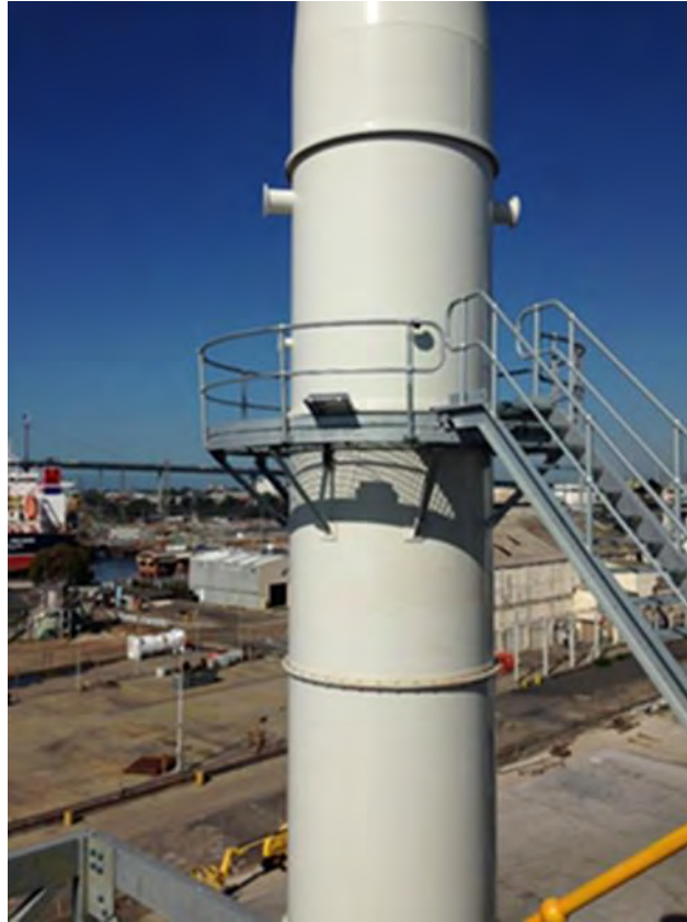
DP1 – Mill Stack
