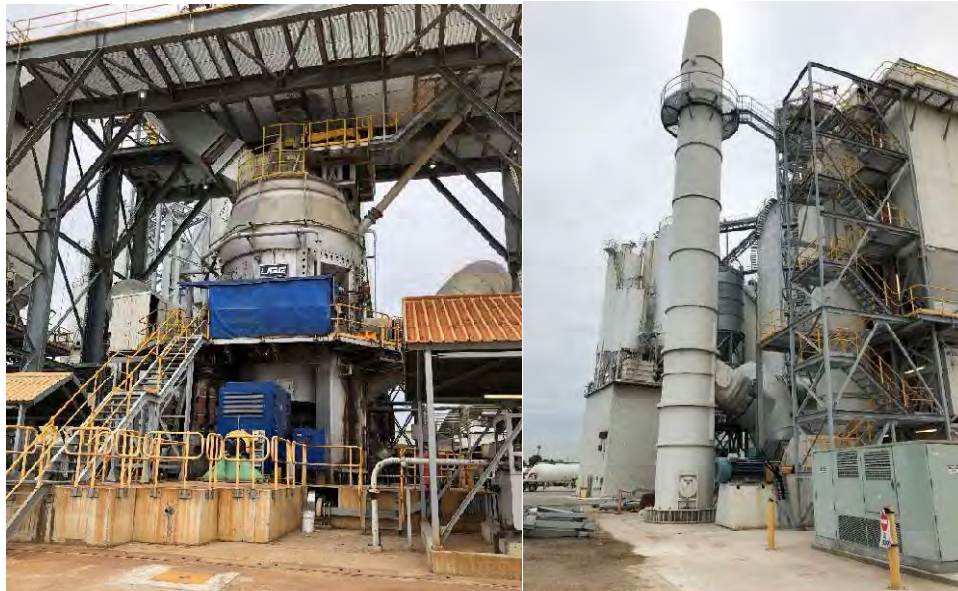
(a) (b) Figure 7: The existing (a) slag grinding mill plant and (b) baghouse stack.
