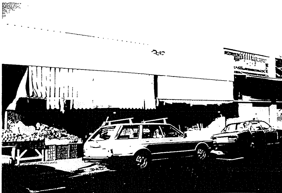
45. SUNBLINDS ILLUSTRATING PROBLEMS WITH MAINTENANCE AND HAZARD TO PEDESTRIANS.
