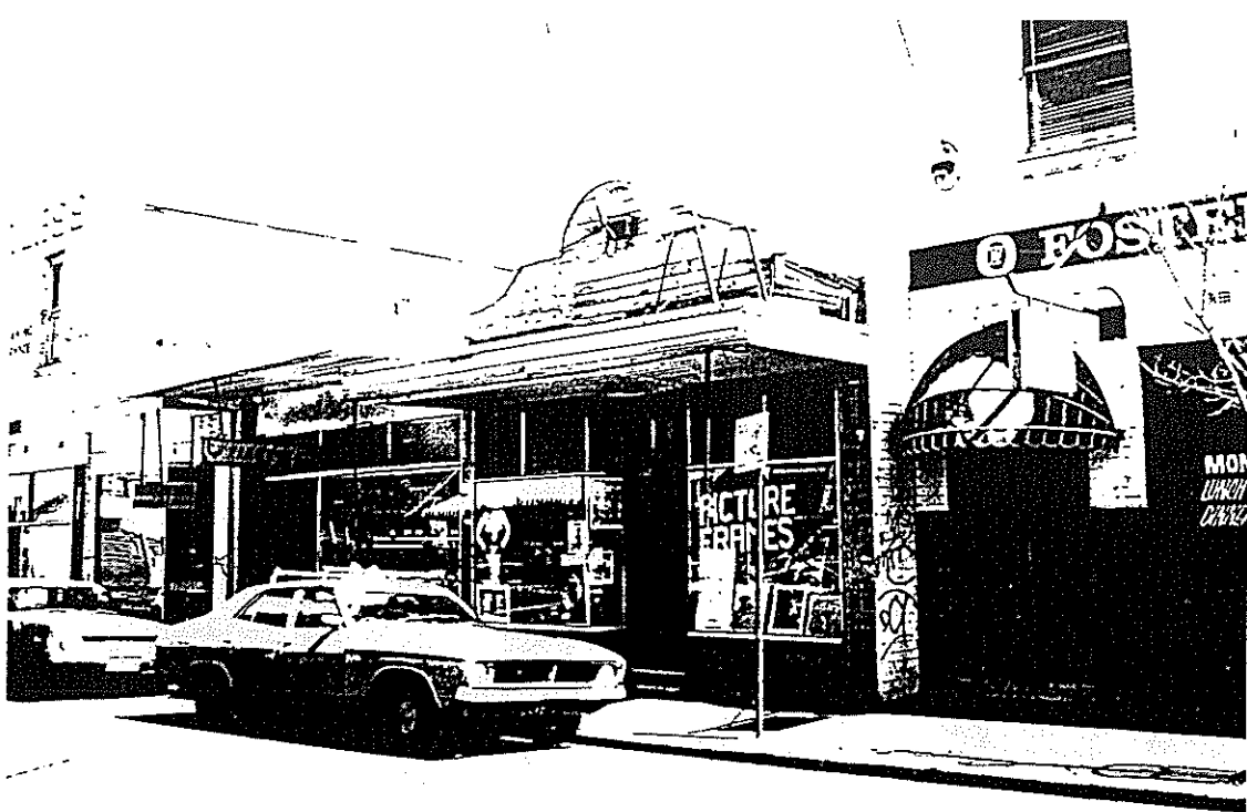
44. LATER CANTILEVERS BADLY FITTED TO EXISTING EARLY BUILDINGS.
