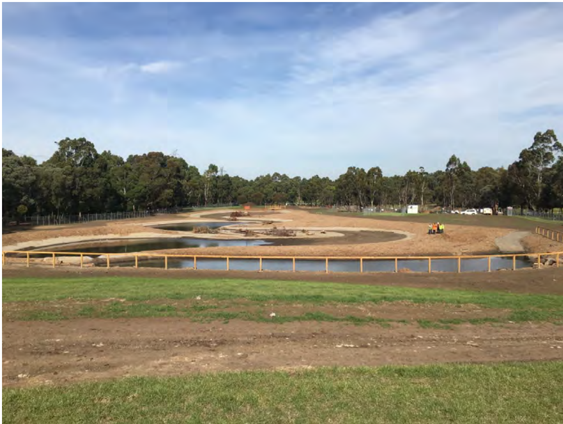
Figure 3 Alluvium/Rakali designed wetland recently constructed in 2016
