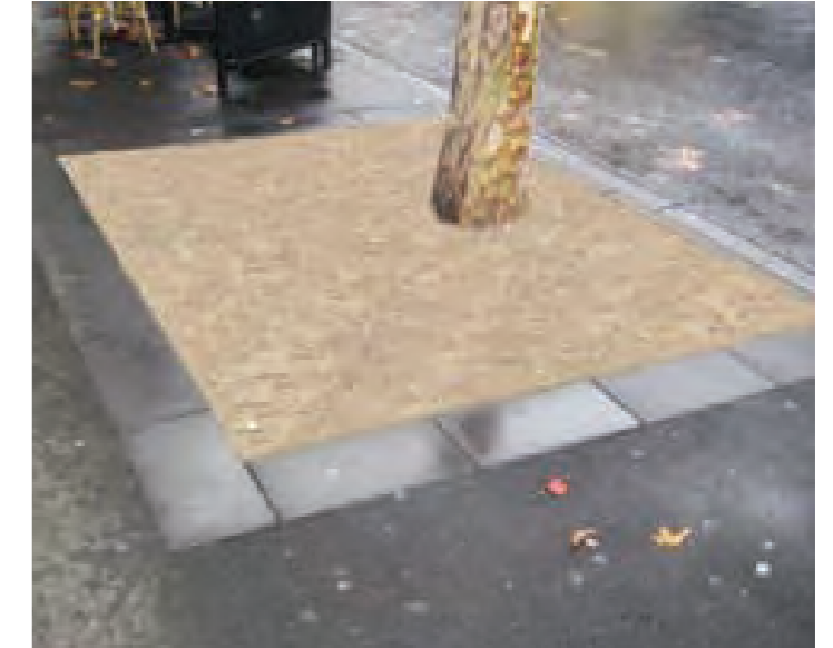
Tree Surround in Footpath
