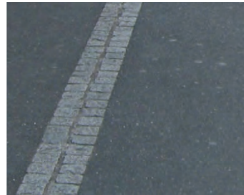
Row of bluestone setts at edge of shared zone
