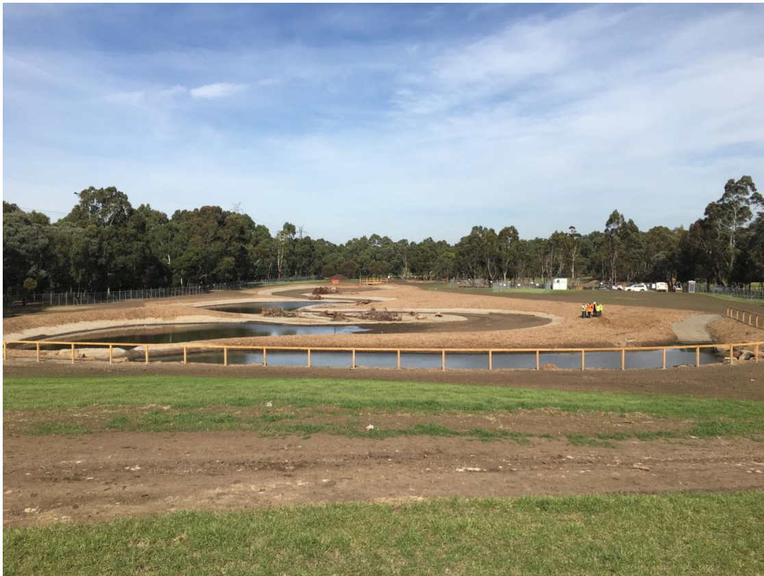
Figure 3 Alluvium/Rakali designed wetland recently constructed in 2016
