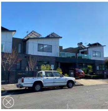
Roof design that does not consider provision of solar panels can result in a disjointed outlook.
