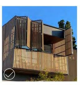
Doors, windows and balconies facing east and west should consider integrated external shading devices to provide greater sun control for the occupants in various seasons.
