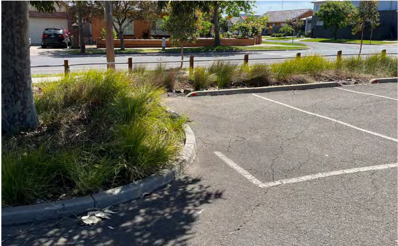
Carpark cutouts and swales, West Footscray
