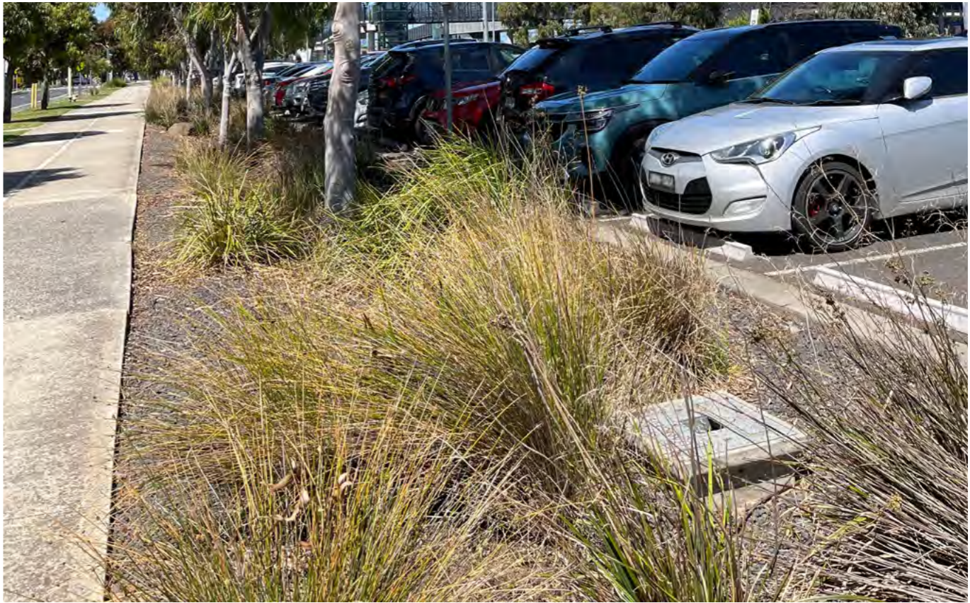
Carpark cutouts and swales, West Footscray
