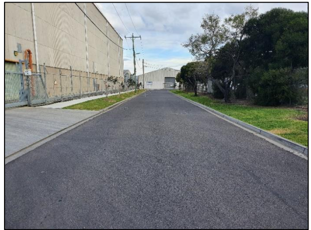
Figure 7: Stradbroke Street – View South
