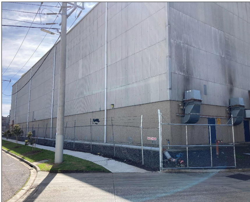
Figure A2 Watty Facility Building Forced Extraction Vents
