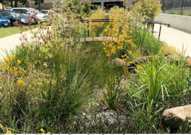
Water Sensitive Urban Design: Dawson Street Precinct, Sunshine Urban swales treat stormwater runoff and provide opportunities for planting, feature lighting and play. This swale includes two pedestrian bridges and rocks allowing kids to jump across
