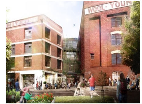
Adaptive restoration and re-use underway of the Young Husband Woolstores in Kensington as an industrial village https://www.younghusbandwoolstore.com.au/the-vision
