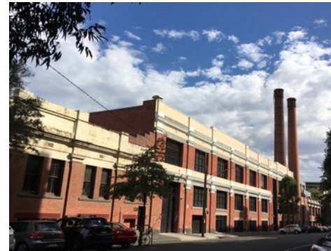
Adaptive re-use of the Foy and Gibson Factory Buildings, Collingwood for a range of light industry and office ©GJM Heritage
