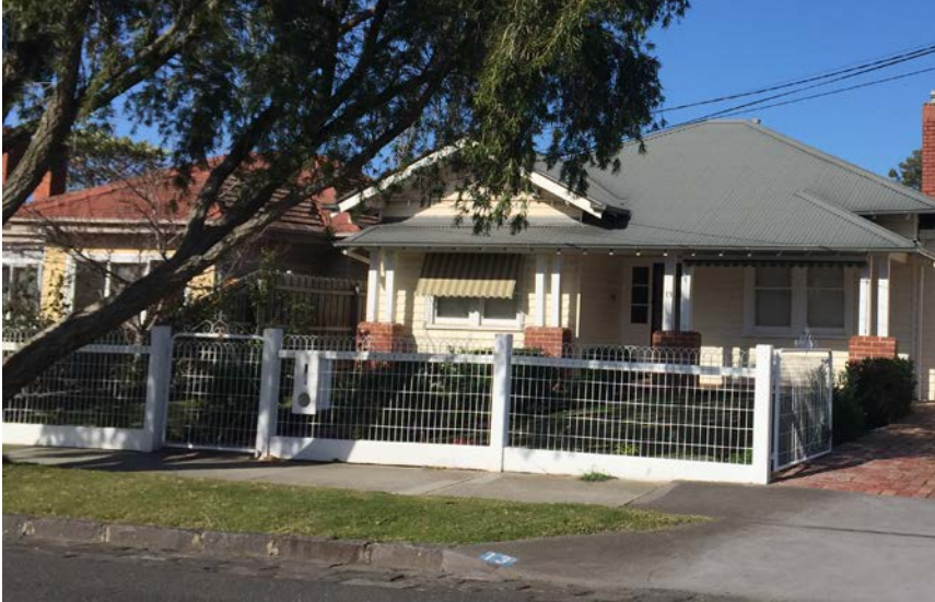
Figure 12 Replacement timber-posted woven wire fencing, HO12 War Service homes heritage area Maribyrnong
