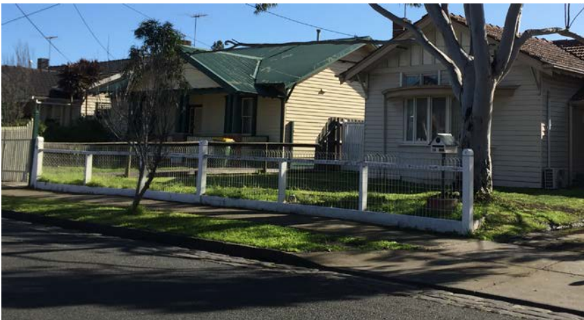
Figure 11 Original timber-posted woven wire fencing, HO12 War Service homes heritage area Maribyrnong
