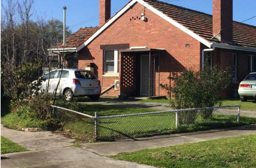
Figure 10 Original low steel and cyclone wire fence, HO5 Munitions worker's housing heritage area Braybrook
