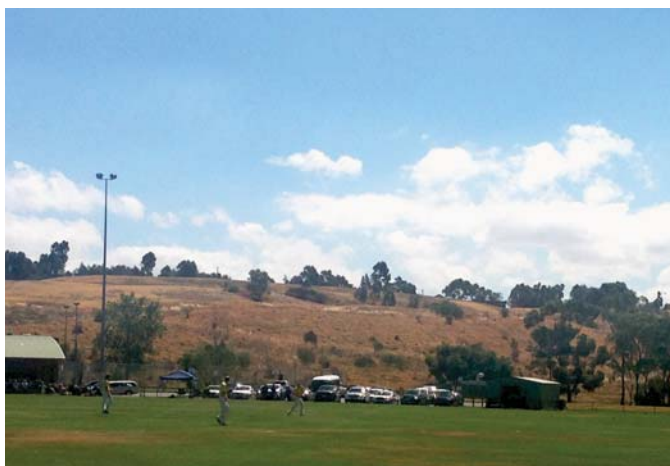
4 View of site from east
